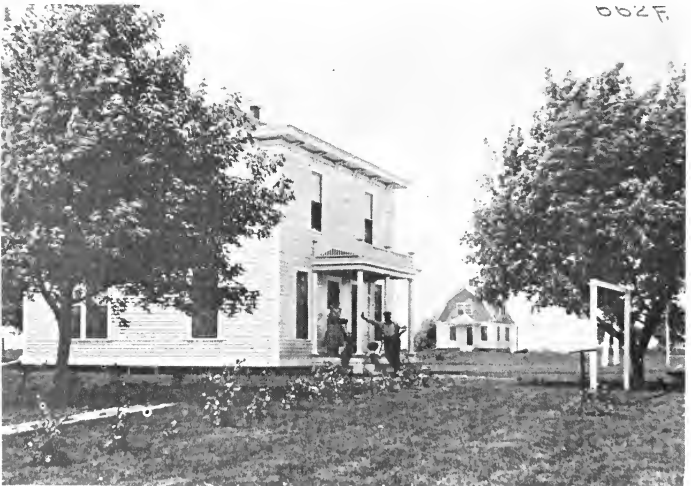
Overseer's and locktender's houses at Lock 22. (Photograph courtesy of Hennepin Canal Parkway )
